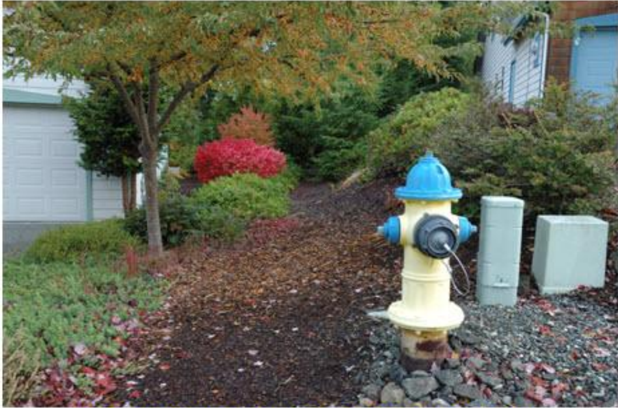
Photo 5 between lots 25 & 26 on Leighbrook Ln.
